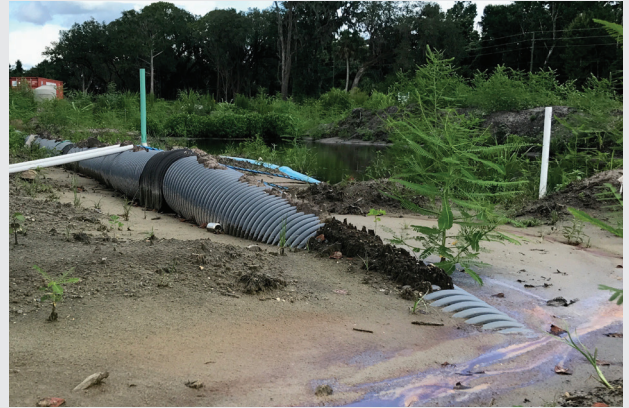
18-inch diameter polypropylene pipe flotation at residential subdivision project in the City of Winter Springs, 2018.
