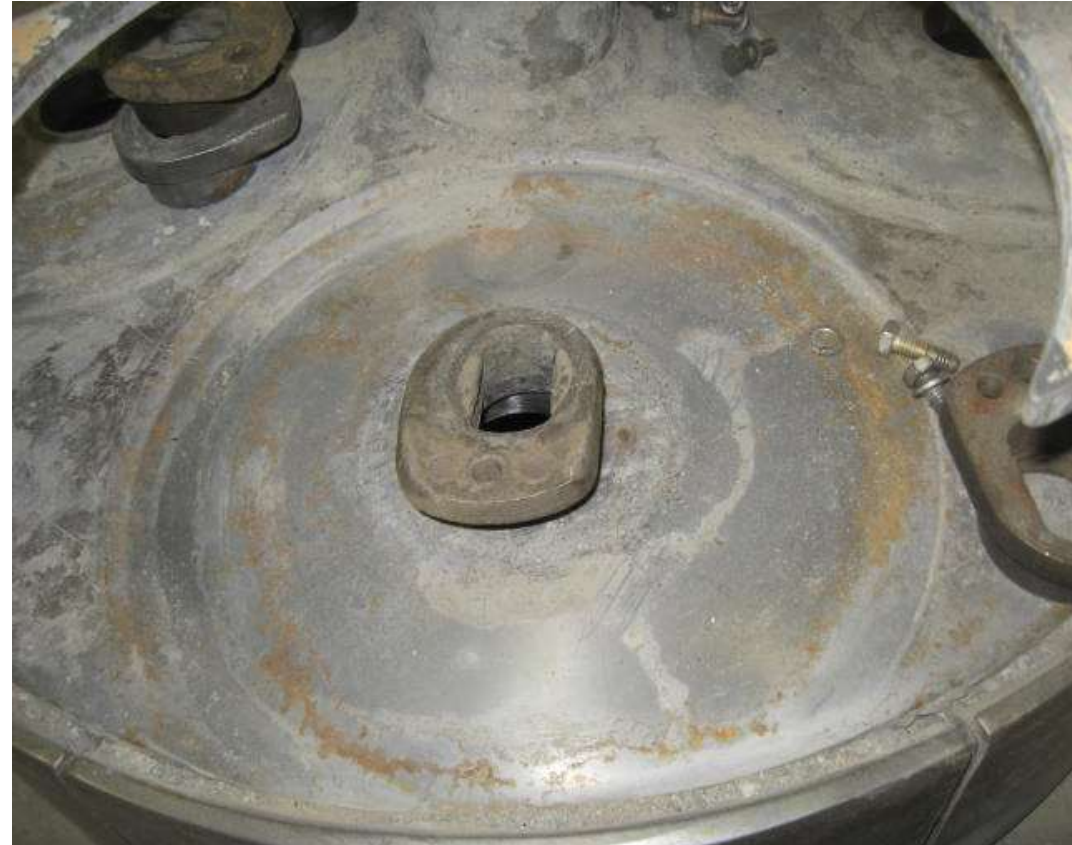
Worn rollerhead frame
