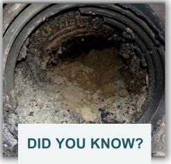
When plastic pipe burns and melts, it--and the roadway above it--must be replaced. The drainage culvert is unusable until the replacement is made. This affects the environment and community while increasing the risk of flooding.
