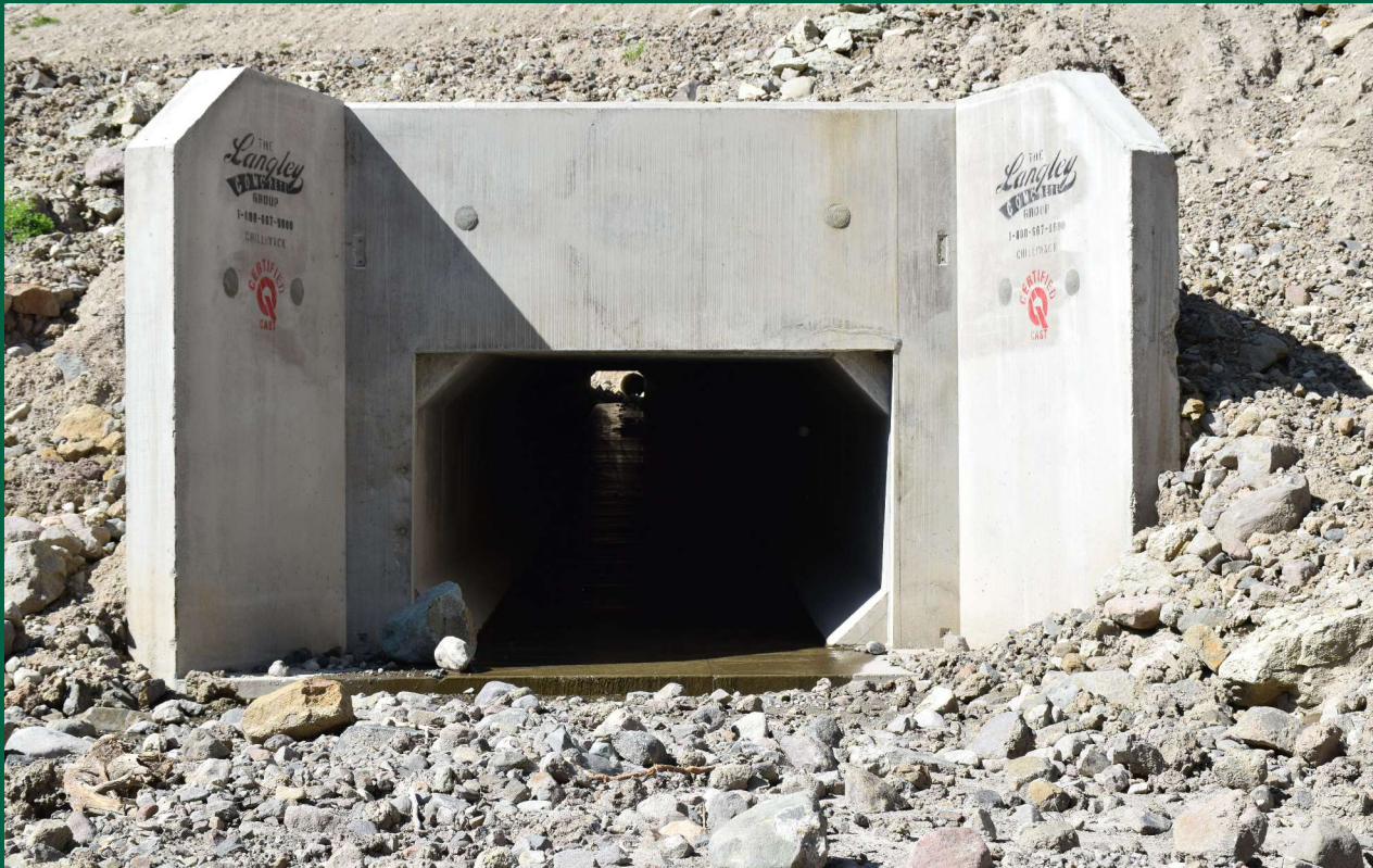
Langley Concrete Group delivered precast concrete box culvert and headwall structures from its QCast-certified operations for a British Columbia Ministry of Transportation contract aimed at improving road safety and drainage system capacity.
