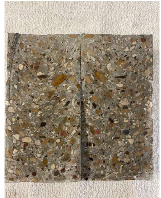
No VMA Aggregate at top No Segregation
