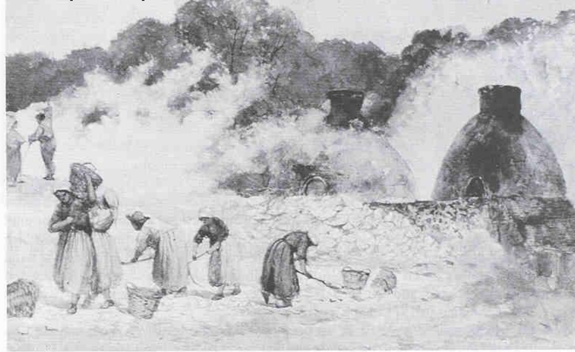
Fig. 1.3 Joseph Aspdin's first cement works at Kirkgate, Wakefield (ca 1828); proto-Portland cement was manufactured at this plant.
