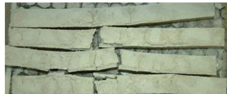
Fig. 8-8. Example of sulfate attack in concrete.
