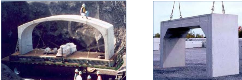
Fig. 1-20. Examples of three-sided / u-shaped concrete structures.
