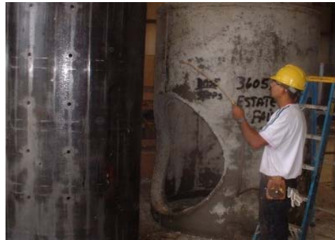
Figure 2-8. Illustration showing the application of the form release agent.
