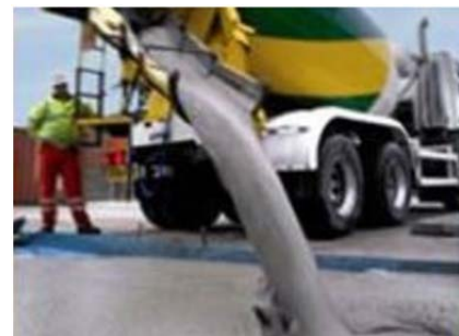
Fig. 7-9. SCC delivered in ready-mix
