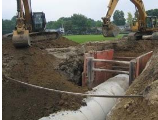
Fig. 8.1.concrete pipe installation
