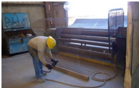
Fig. 1-6. Wire roller used in wire cage fabrication.
