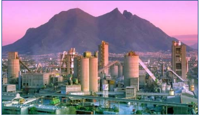
Figure 2-1. Cemex, Monterrey, Mexico.
