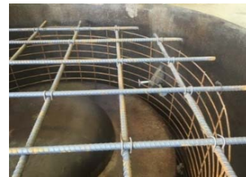
Fig 1-11. Typical manhole base section reinforcement.
