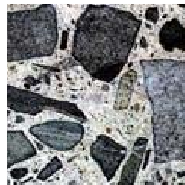
Fig. 8-7. Cracking within aggregates in reactive carbonate aggregates surrounded by high-alkali cement.
