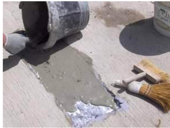
Fig. 2-10. Illustration of a bonding agent being applied to concrete defect area.
