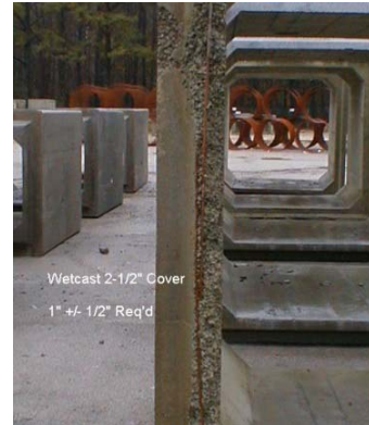
Fig. 1-9. Illustration of a damaged end that should be rejected.
