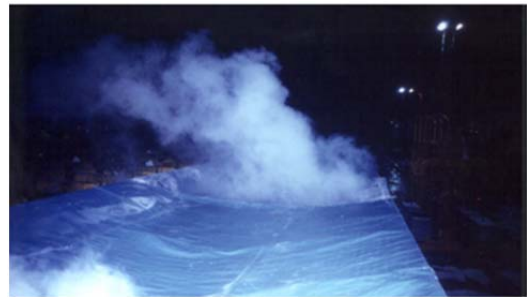
Fig 4-5. Illustration of flueing--the problem of energy and steam being released out the top.
