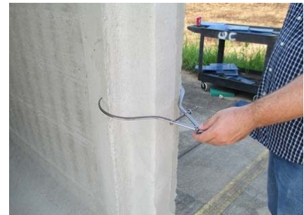
Fig. 1-7. Conducting a dimensional check on a box culvert using measurement calipers.
