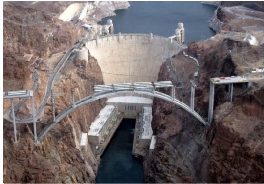
Fig. 1-1. The Hoover Dam, Boulder City, NV, USA.
