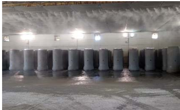
Fig. 4-2. Illustration of a fogging/misting system.
