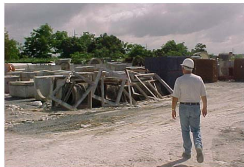
Fig. 2-4. Illustration of improper storage.
