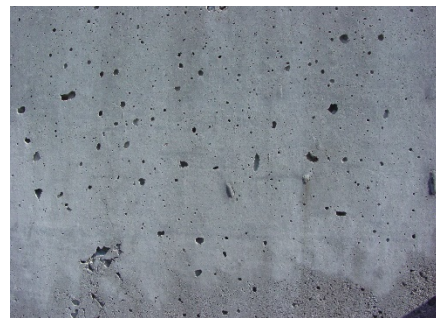
Fig. 3-5. Illustration of bugholes in
