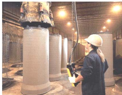
Fig. 1-2. Illustration of stripping forms from concrete pipe.
