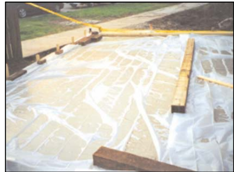
Fig. 4-3. Illustration of polyethylene film being used as an effective moisture barrier during concrete curing.
