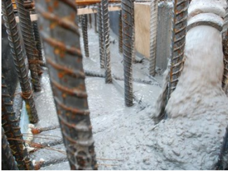
Fig. 7-10. SCC easily flows around obstructions with no vibration. Joe Woolhead for iCrete.
