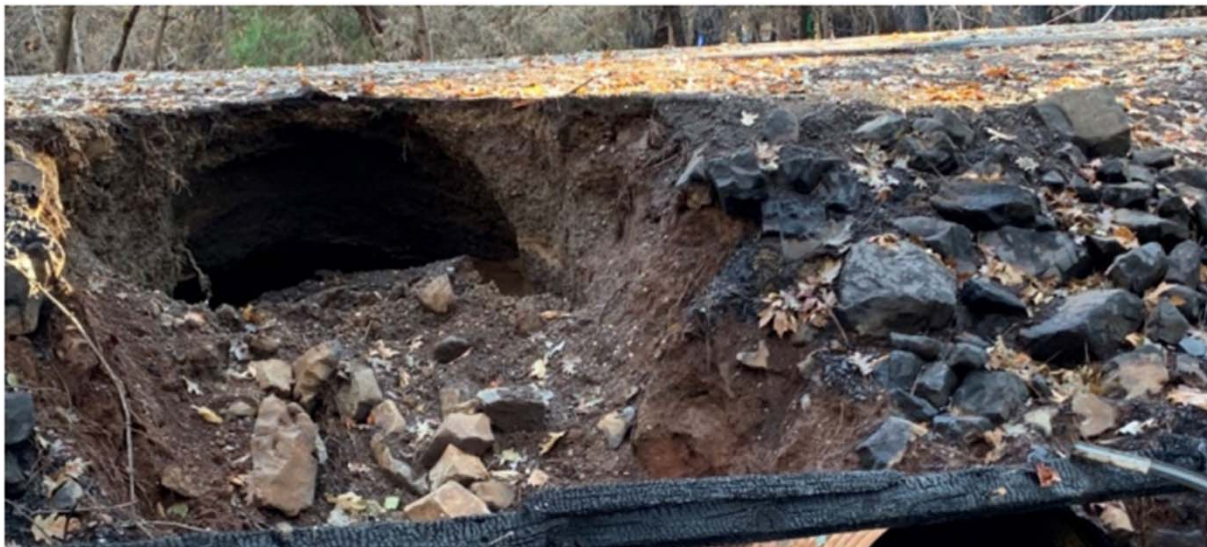
Figure 4 - Collapsed Culvert on Roe Road
