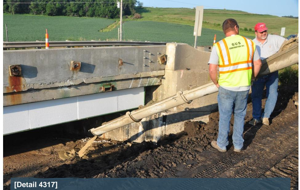
"construct earthfill soil plug beyond limits of deck width... fill void with the maximum amount of floodable backfill possible... distance from floodable backfill to bridge beams shall not exceed 5'... place Stage 1 flowable mortar to within 6" of bottom of beams."
