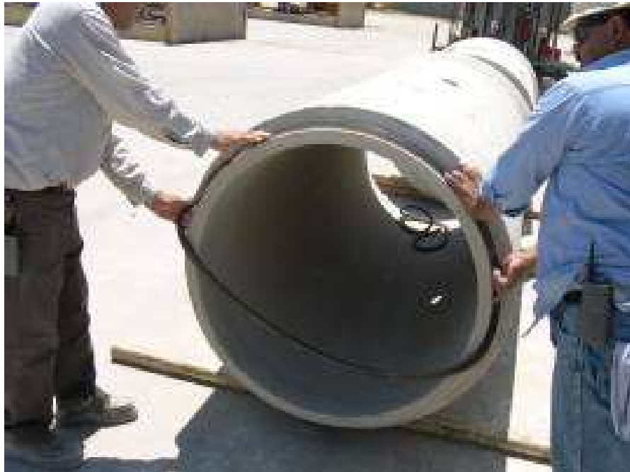
Mount gasket on dry spigot
