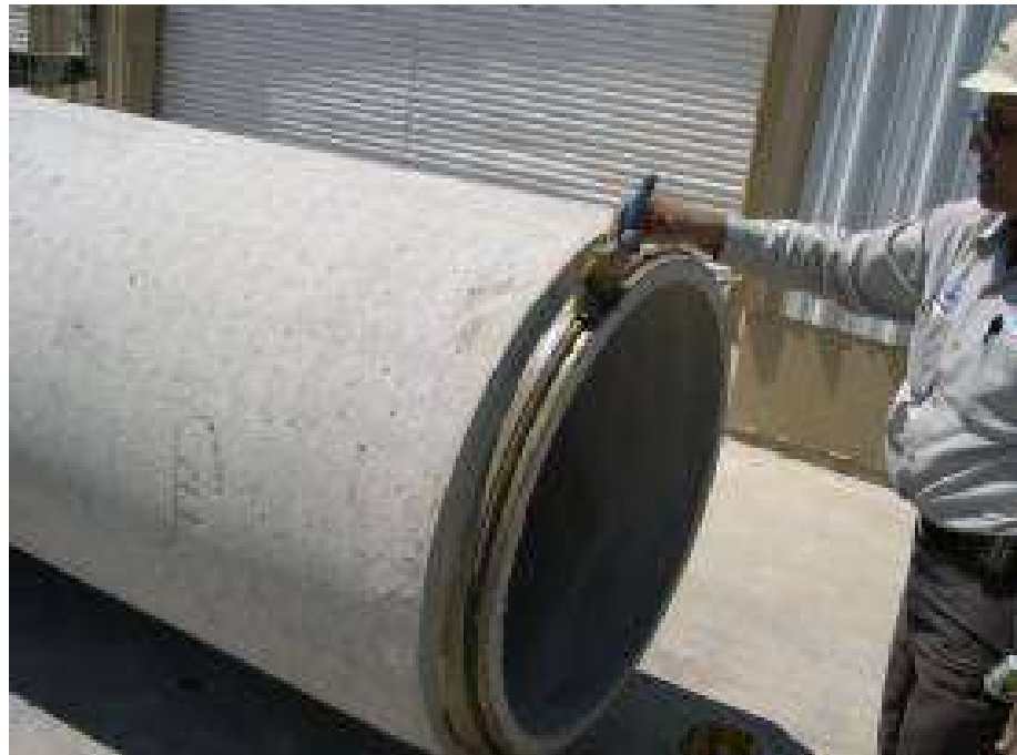
Lubricate exterior surface of gasket
