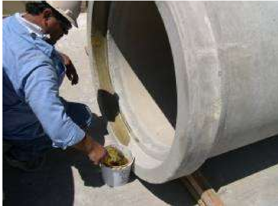
Lubricate bell surface
