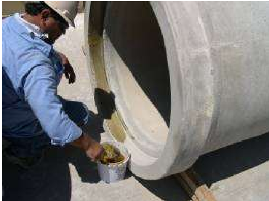
Lubricate the bell
