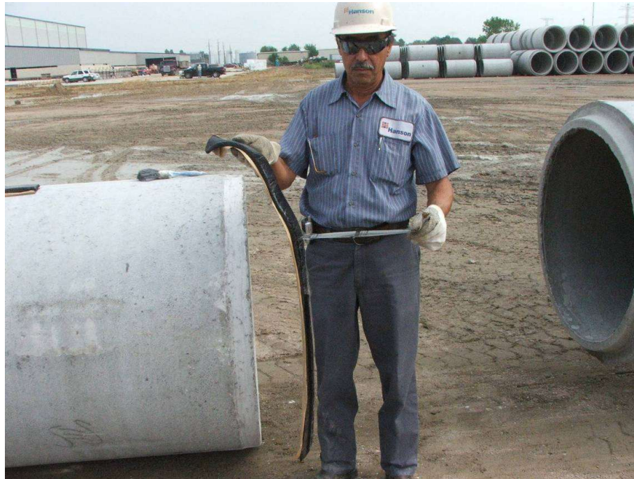
Remove cover from one side of Preformed Mastic Gasket piece
