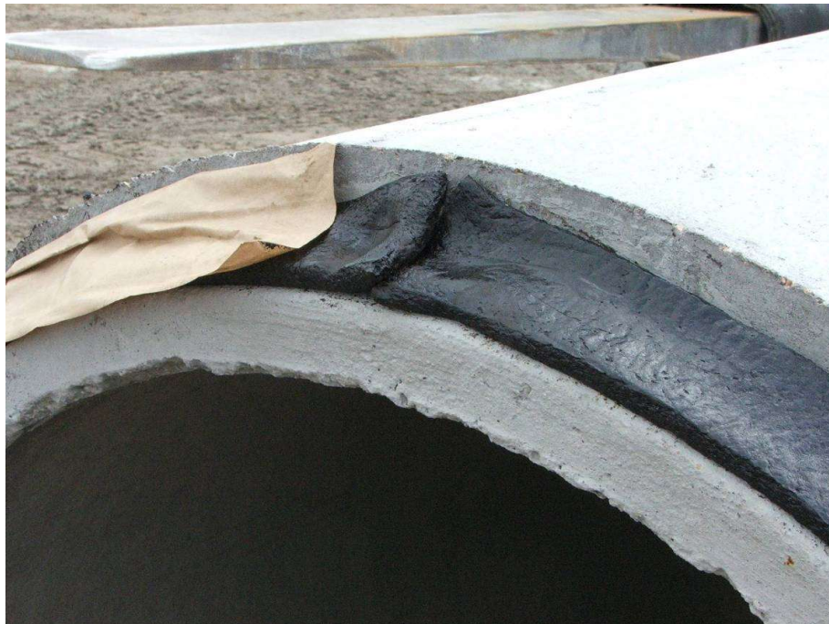
Butt Mastic pieces to splice
