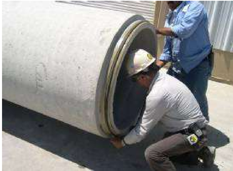
Mount gasket on spigot
