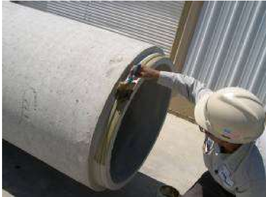
Lubricate spigot surface and gasket groove
