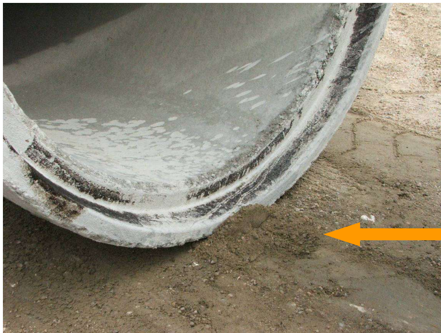
T&G or RG Pipe – This will keep joints from closing evenly
