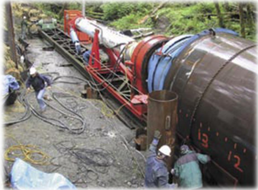
Pipe Ramming to install a parallel pipe (upstream and downstream)
