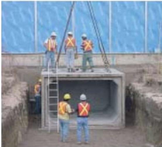
*The precast concrete box sections were installed on a "mud slab." Sand bedding was placed over the*
