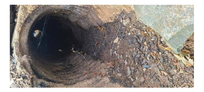
As a wind-driven fire with low-flying embers, miniature fires were ignited inside open-ended culverts and, depending on the construction material type, completely burned out several pipes, collapsing and undermining the ROADWAY...
