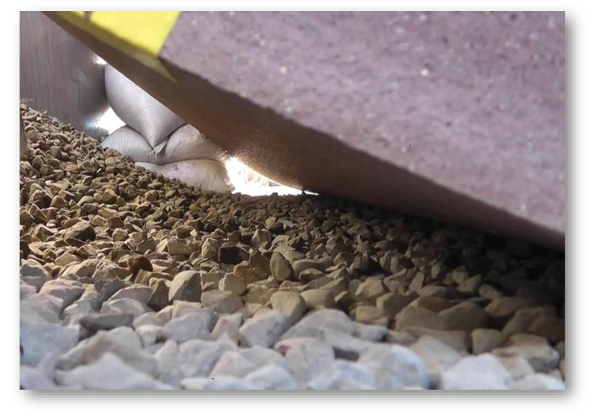
CONCRETE PIPE BEDDING FACTORS FOR EMBANKMENT INSTALL – IN THE DESIGN CODE – WERE ADJUSTED TO ACCOUNT FOR VOIDS IN HAUNCH.
